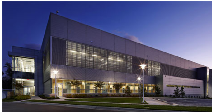
(a) NetApp Data Center in RTP
