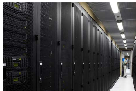
(e) Server Rooms
