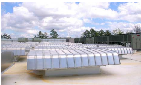
(b) Air inlet units
