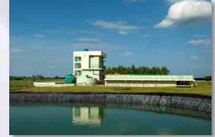
Water & Sewage Treatment
