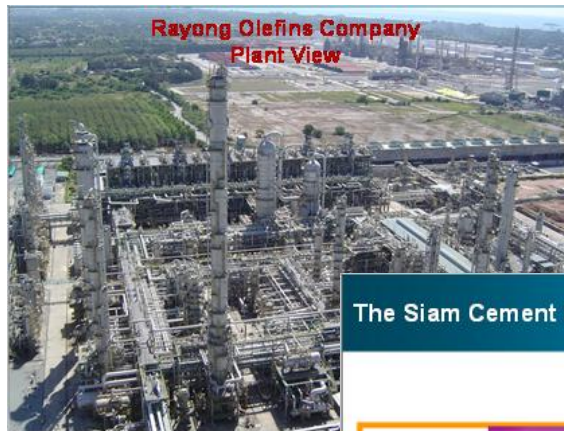
Fig-1: ROC plant view
